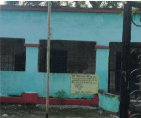
Polling Station Front View
