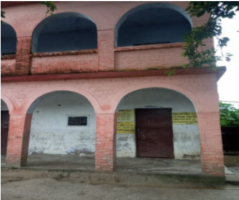
Polling Station Building Front View
