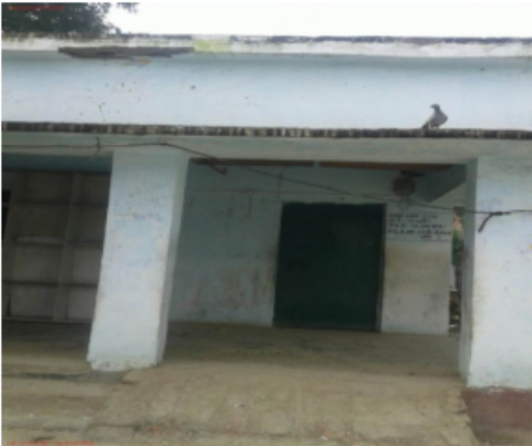
Polling Station Building Front View
