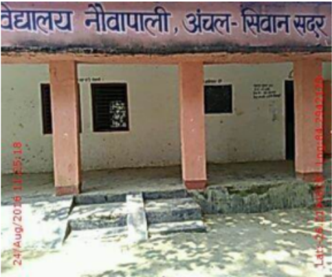
Polling Station Building Front View
