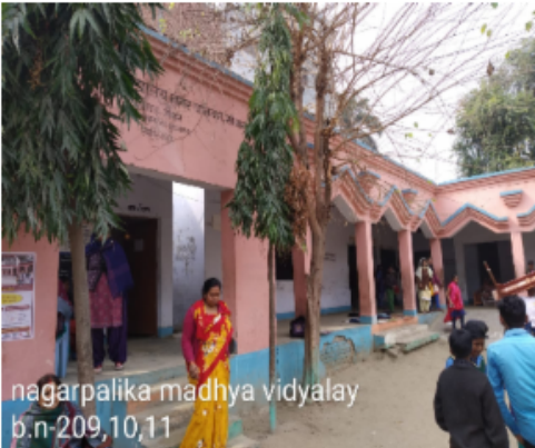
Polling Station Building Front View
