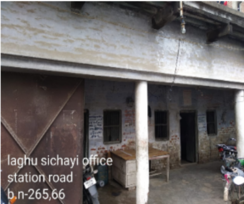
Polling Station Building Front View
