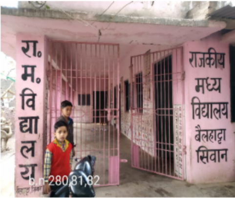
Polling Station Building Front View
