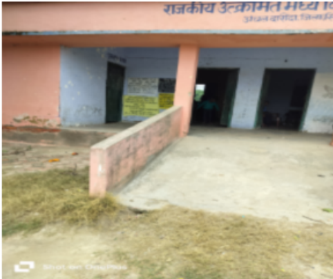
Polling Station Front View
