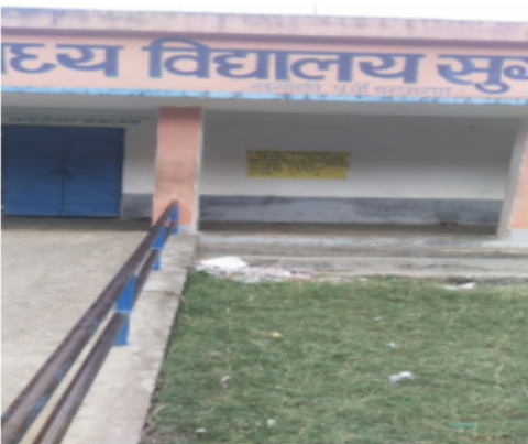
Polling Station Front View
