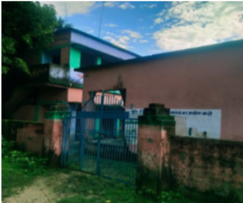
Polling Station Front View
