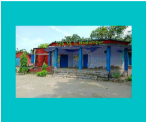
Polling Station Front View
