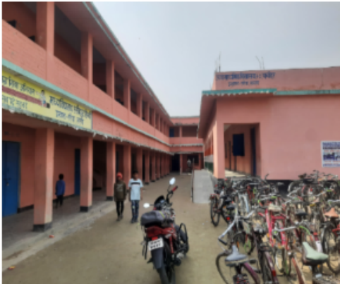
Polling Station Front View
