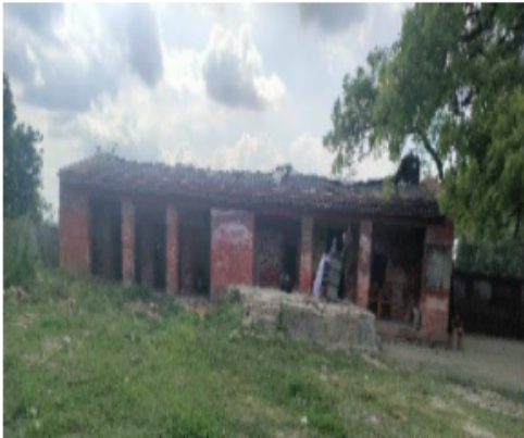
Polling Station Front View
