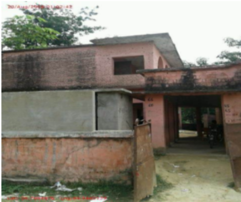
Polling Station Front View
