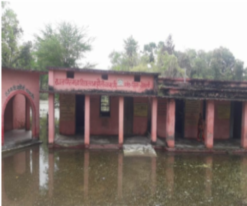
Polling Station Front View
