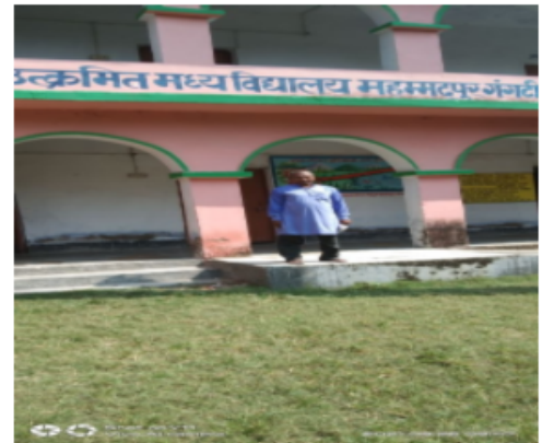
Polling Station Front View
