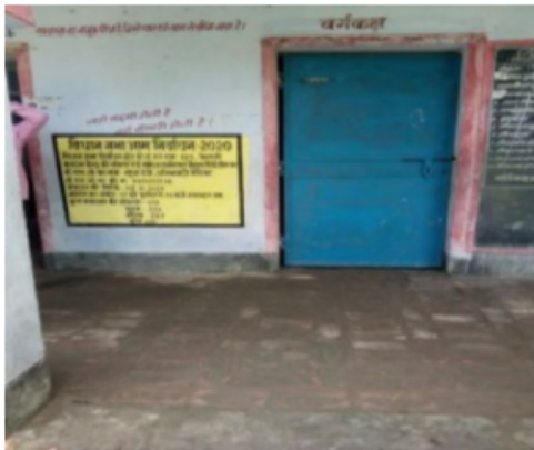
Polling Station Building Front View
