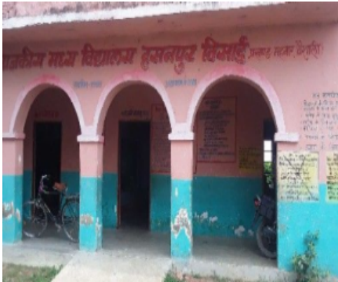
Polling Station Building Front View
