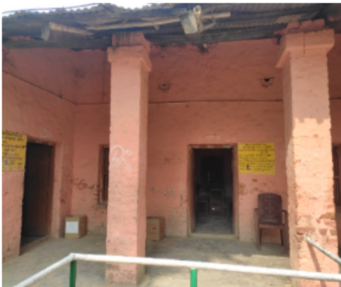
Polling Station Front View
