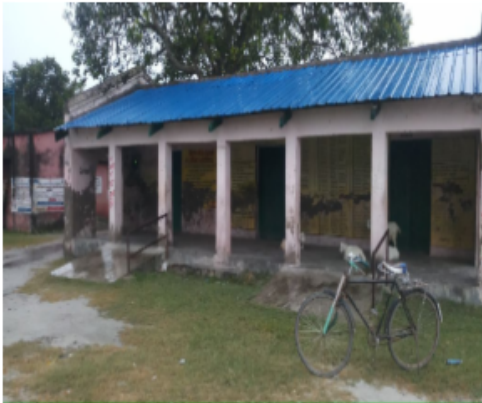
Polling Station Front View
