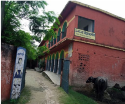
Polling Station Front View
