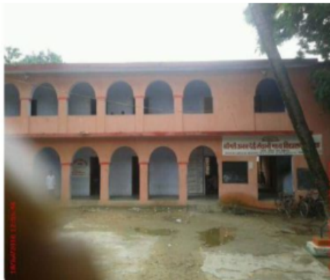
Polling Station Building Front View
