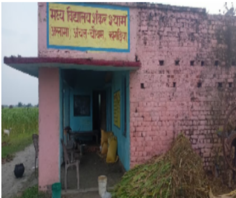
Polling Station Front View
