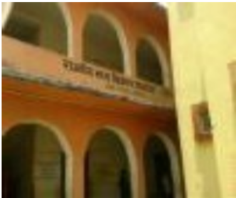
Polling Station Building Front View
