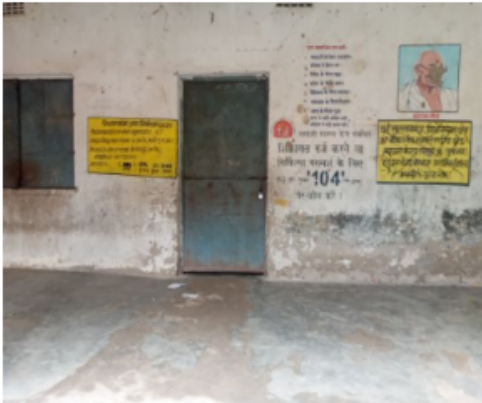
Polling Station Front View
