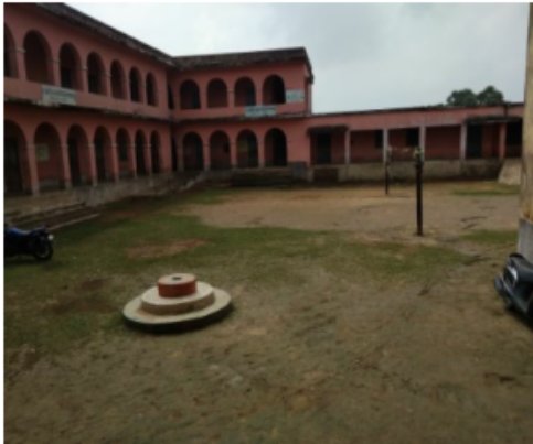
Polling Station Building Front View
