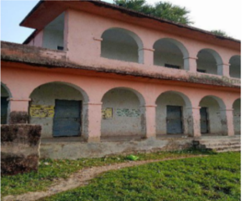
Polling Station Front View
