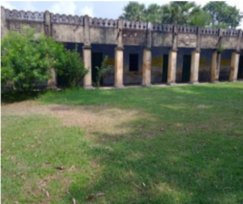
Polling Station Building Front View
