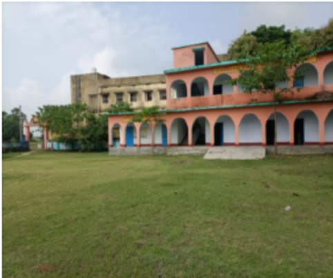
Polling Station Front View
