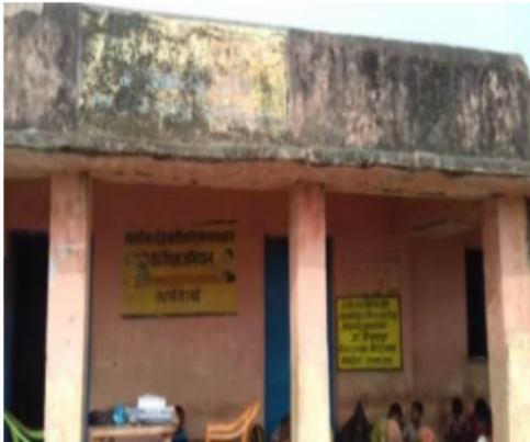
Polling Station Building Front View
