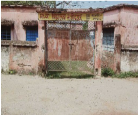
Polling Station Building Front View
