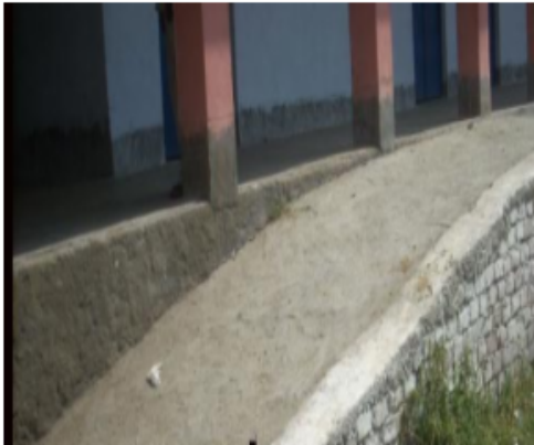
Polling Station Building Front View
