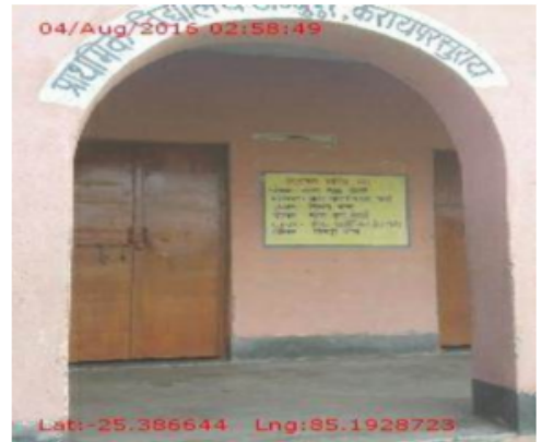
Polling Station Front View
