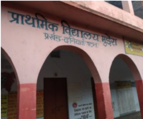
Polling Station Front View
