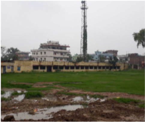
Polling Station Front View
