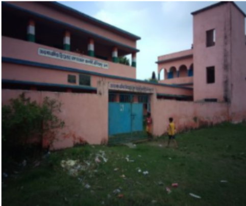
Polling Station Front View
