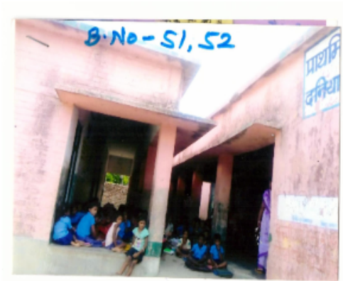
Polling Station Front View
