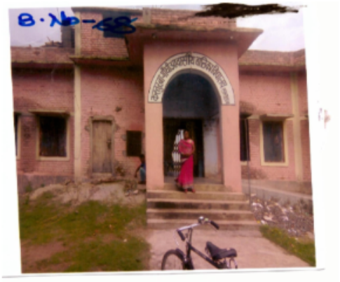
Polling Station Front View
