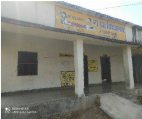
Polling Station Front View
