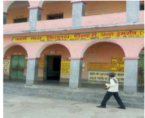
Polling Station Front View
