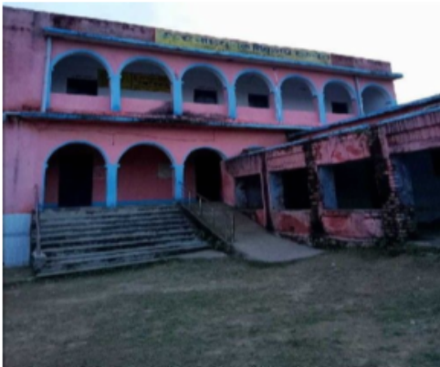
Polling Station Front View
