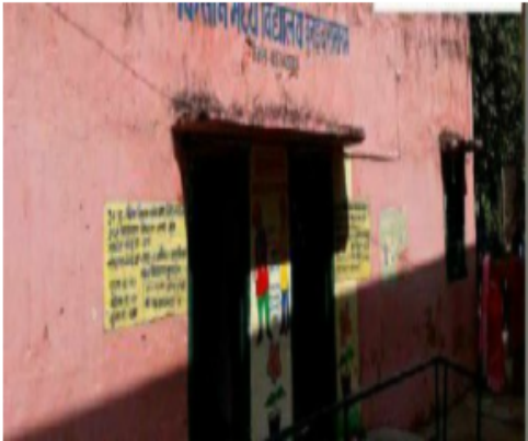
Polling Station Front View
