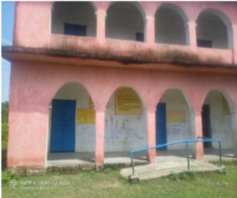
Polling Station Front View
