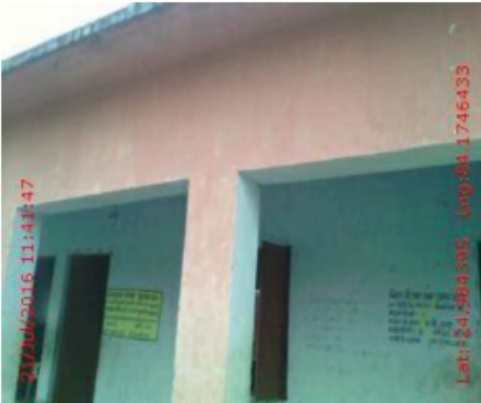
Polling Station Building Front View
