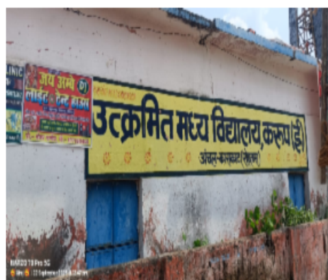
Polling Station Front View
