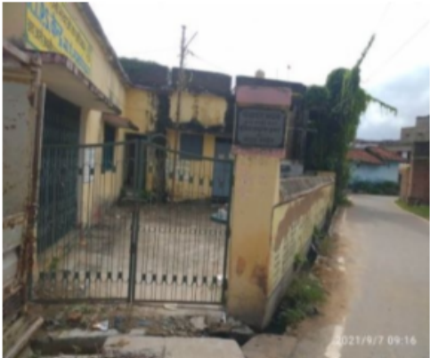
Polling Station Front View
