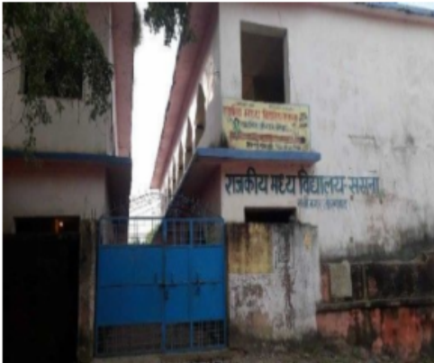
Polling Station Front View
