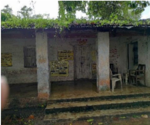
Polling Station Front View
