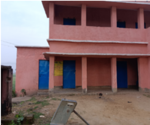
Polling Station Front View
