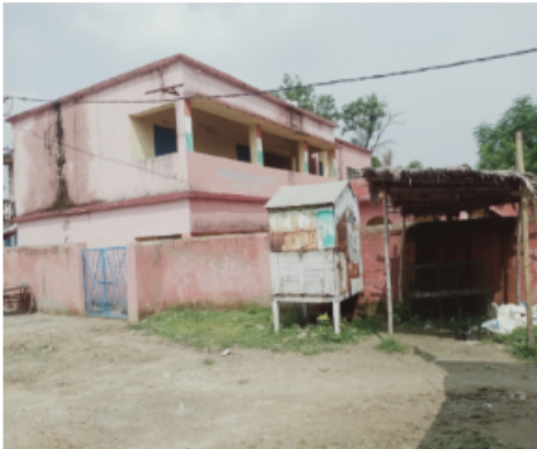
Polling Station Front View
